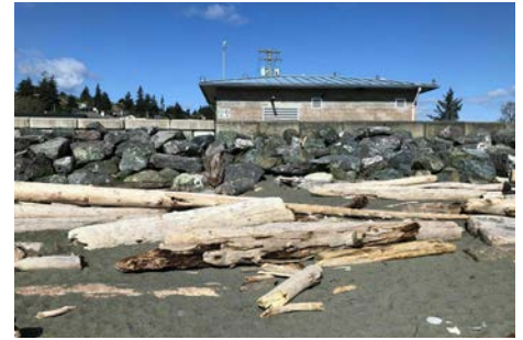
Beach Armoring at the Pump Station
