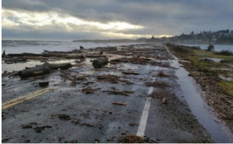
Winter Storm Debris on Ocean Boulevard Source: Linda Gower
