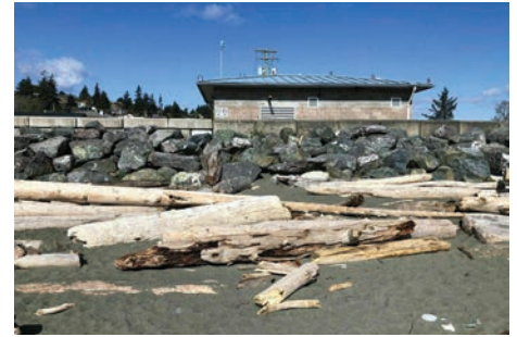
Beach Armoring at the Pump Station
