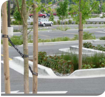
An example of a parking area with bio-swales for rainwater infiltration.
