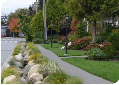
An example of how a residential street can incorporate rain gardens to capture stormwater from impermeable
