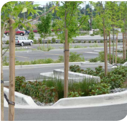
An example of how a surface parking lot incorporates rain gardens.
