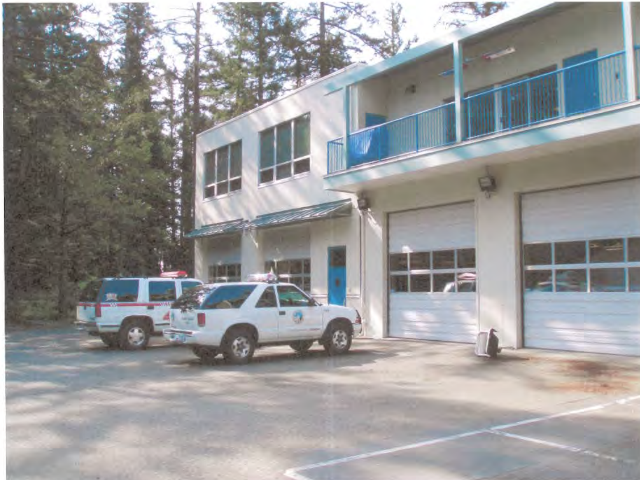
Colwood Fire Hall
