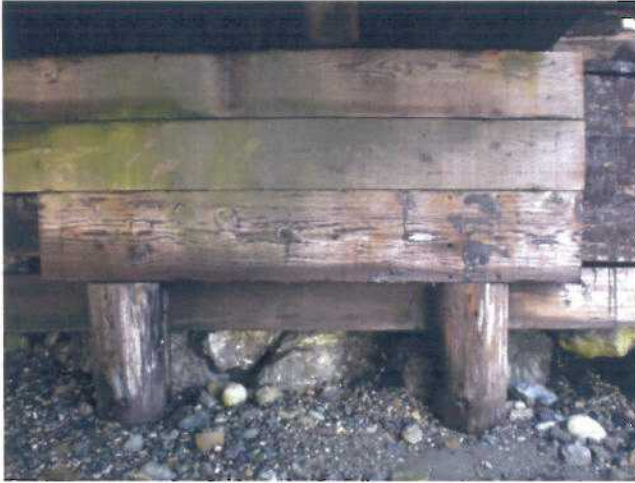
P10 - North Abutment face - seaward side below edge of deck.
