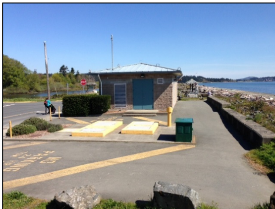
Figure 1-2: Ocean Boulevard Pump Station, wet well in foreground
