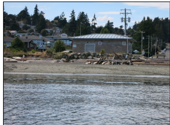
Figure 1-3: Pump Station as seen from the sea
