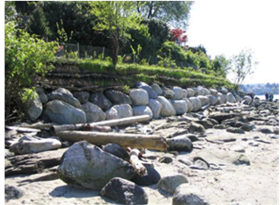
Figure 4-3: Bioengineered Slope Protection
