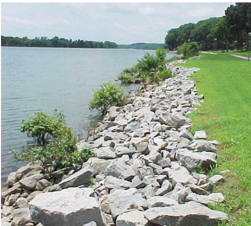
Figure 4-1: Riprap Slope Protection
