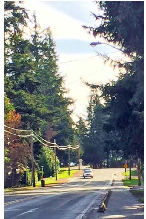
Metchosin Road upgrade area
