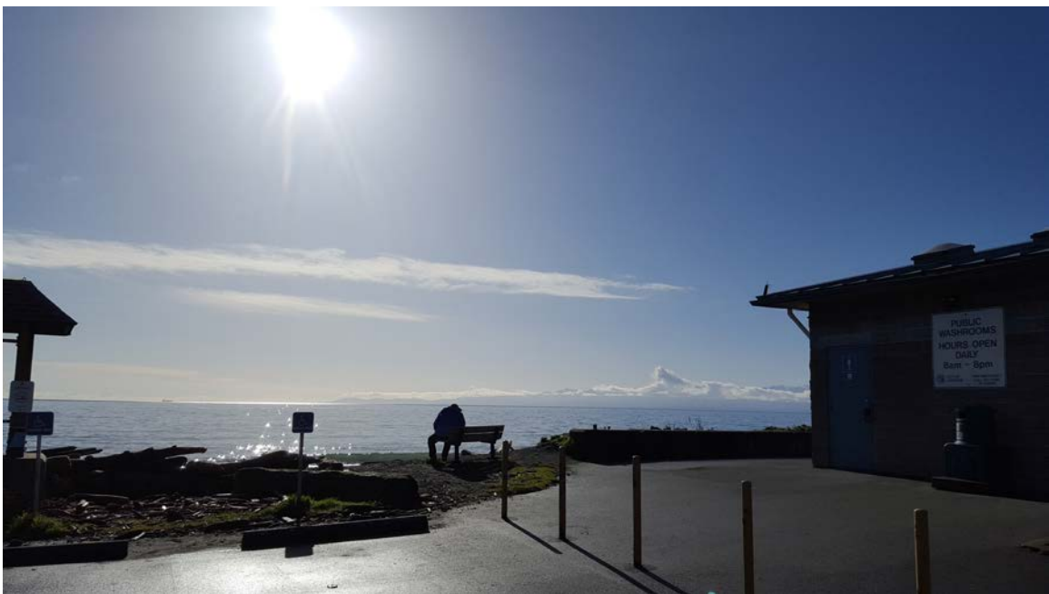
The Lagoon Pump Station (at right)
