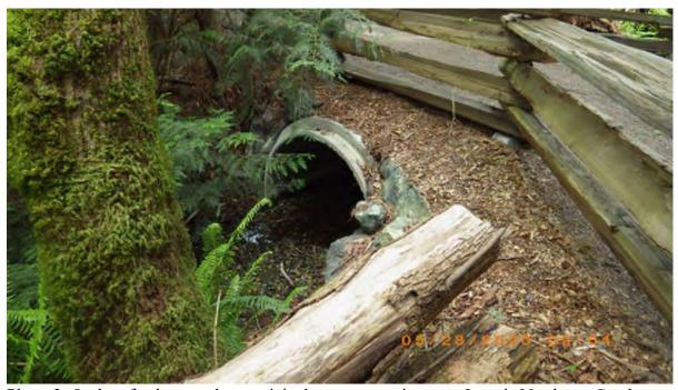
Photo 2. Outlet of culvert under municipal stream crossing over Latoria Northeast Creek.
