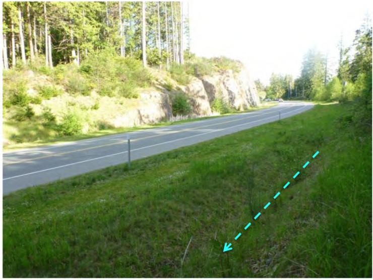
Figure 4. Roadside swale on the east side of VMP. Note there is no evidence of soil or particulate partitioning that would meet the definition of a stream channel within any portion of the bioswale; runoff from VMP appears to consist solely of sheet flow. Dashed line = runoff flow direction. (Photograph taken 2014)
