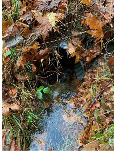
Figure 9. CSP culvert under VMP routing stream flows from the open channel (Figure 8), discharging into Havenwood Creek (Figure 1). Note the clarity of the drainage flow, indicating an absence of sediment transport.
