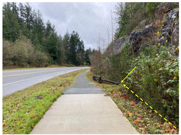
Figure 7. Looking downstream, the yellow arrow points to the drainage flow emerging from the buried drainage channel (dashed yellow arrow). The inlet of this open channel lies within the VMP road ROW adjacent to the northeast corner of the western parcel of the subject property.
