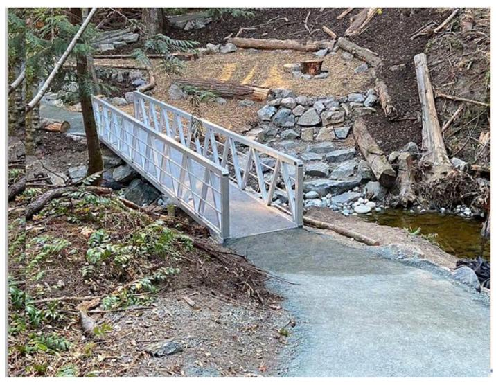
Figure 22. Example of a public walking trail bridge spanning a stream in Mount Douglas Park, Saanich. The bridge is light weight, meets municipal public access, construction standards, minimal maintenance, all-weather, and easily installed (Figure 23). It would be necessary to have a walking surface on the bridge that would be dog-friendly, *i.e.*, not an expanded mesh which could injure the dog's feet.
