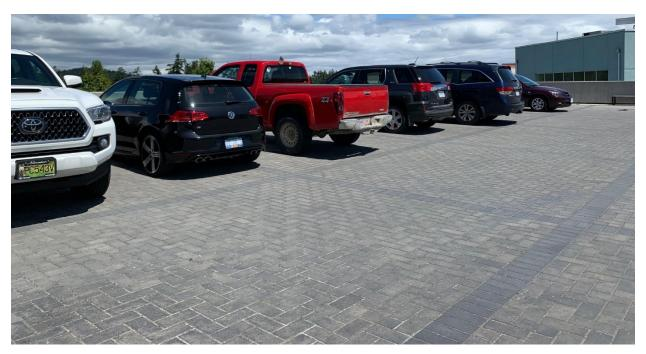
Permeable surface treatment allowing stormwater to infiltrate the sub-surface and contribute less overall run-off to the municipal stormwater system
