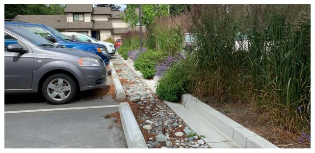
Stormwater management provisions at the foot of the parking space allowing for slower rainwater transport and natural infiltration prior to entering the stormwater system
