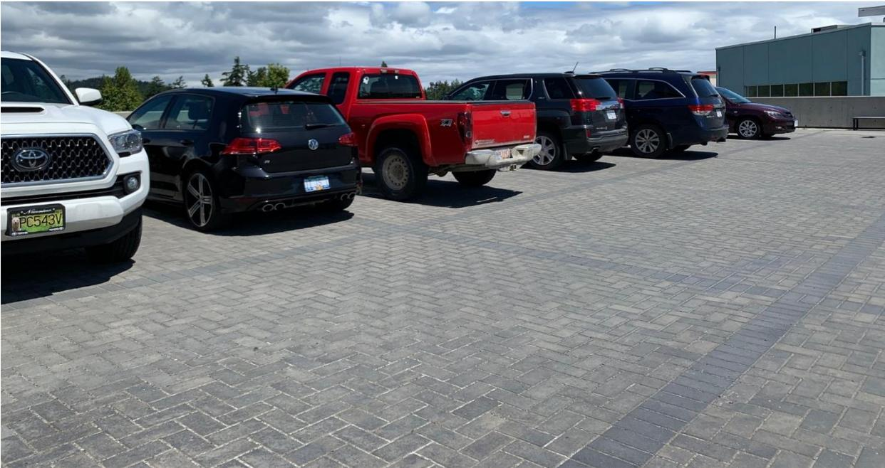
Permeable surface treatment allowing stormwater to infiltrate the sub-surface and contribute less overall run-off to the municipal stormwater system
