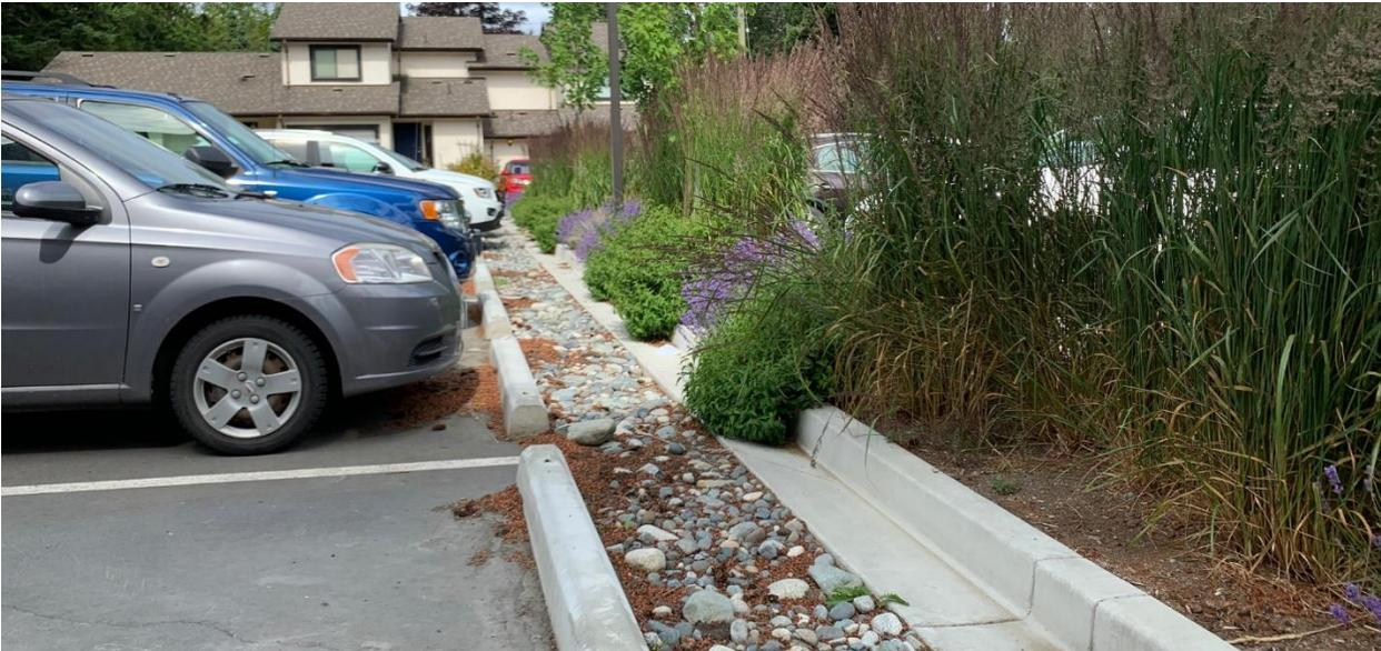
Stormwater management provisions at the foot of the parking space allowing for slower rainwater transport and natural infiltration prior to entering the stormwater system
