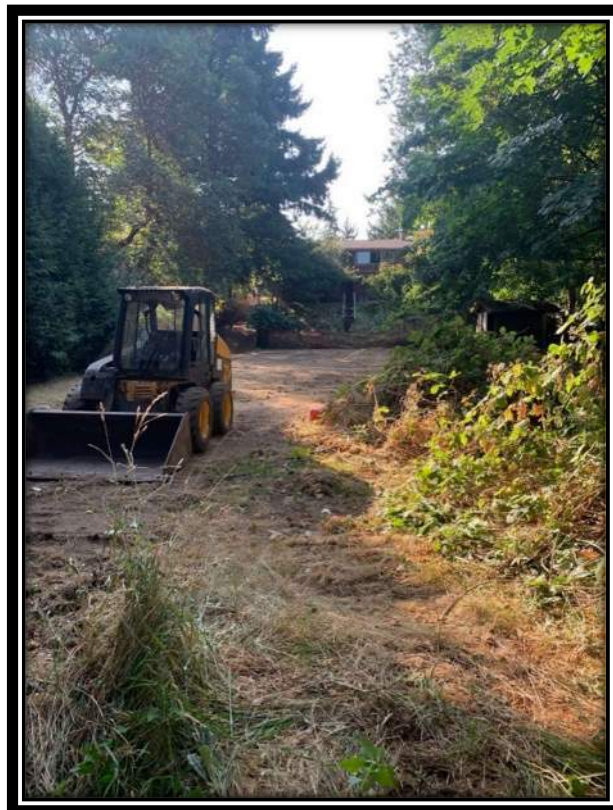
Photograph 8: Looking across backyard from top of slope.
