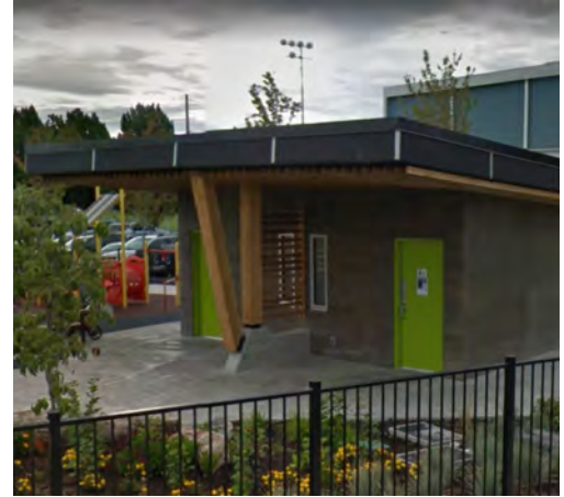
Inspiration: A permanent building with combined washrooms and changerooms is an investment that can add both character and function to Colwood Creek Park.
