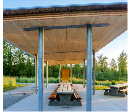
Inspiration: A park shelter structure would provide greater comfort for park users in sun, rain, or snow.
