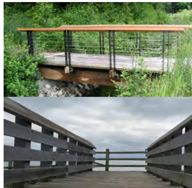
Timber and steel pedestrian bridges
