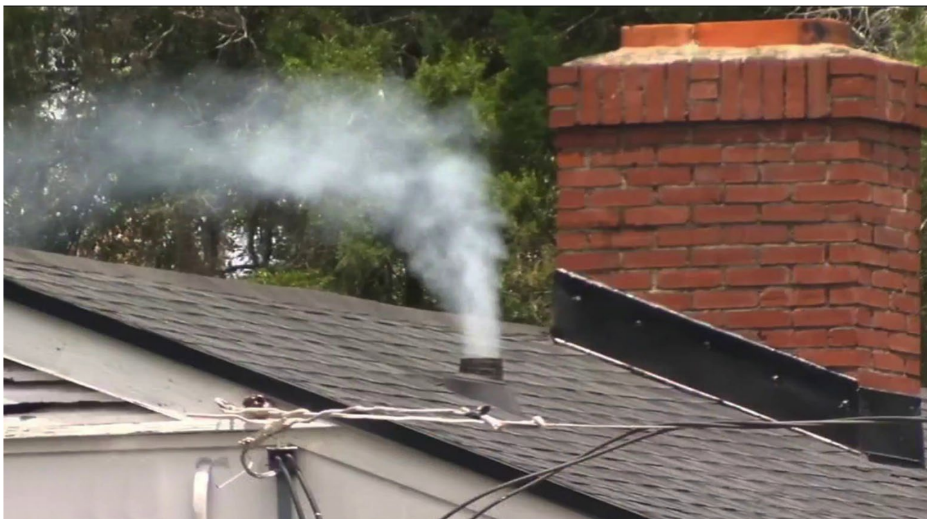
Smoke escaping from a sewer vent (stack) on the roof of a home.
