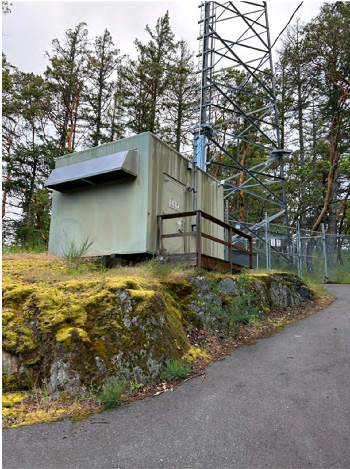
Figure 3- Northwest facing from driveway entrance. Communication structure. Structure and tower to be removed.
