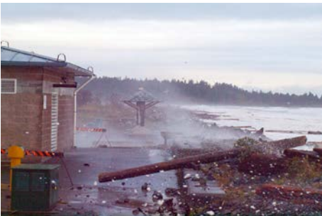
Pump station in a winter storm prior to 2017 berm construction.
