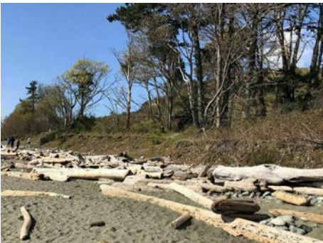
Active Scarp at Perimeter Park
