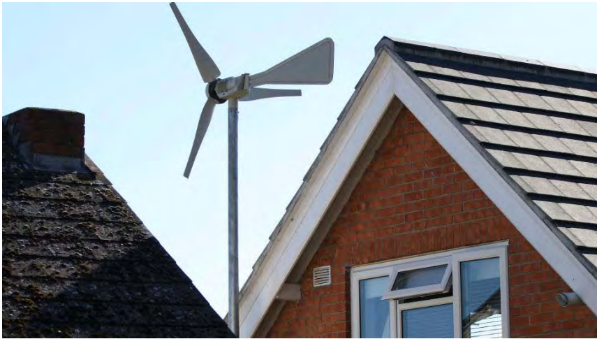
Alternative energy systems
