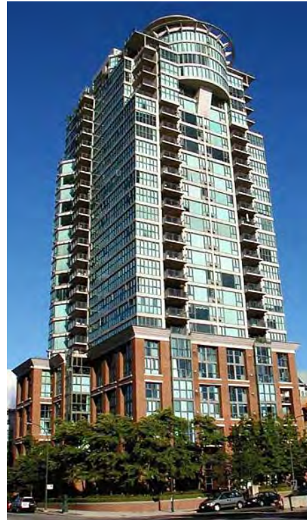
Attractive hi-rise residential buildings
