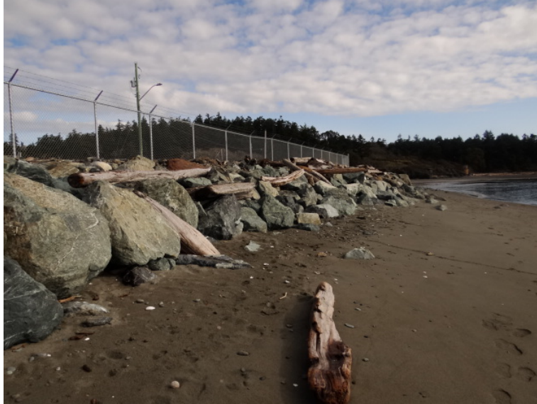
Figure 5. Rip-rap added to the northern end of the peninsula as a mitigation method
