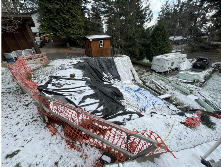
Photo 3. View looking north. All exposed soils have been covered with polyurethane plastic that are subject to rainfall or snow, no evidence of runoff or erosion. January 16,2024
