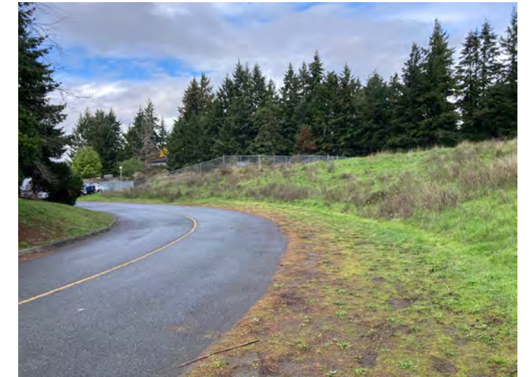
City Hall access road - view to north
