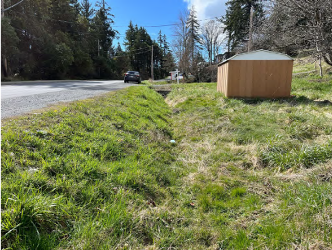
Photo 15. View of ditch from north boundary looking southwest. April 4, 2023.
