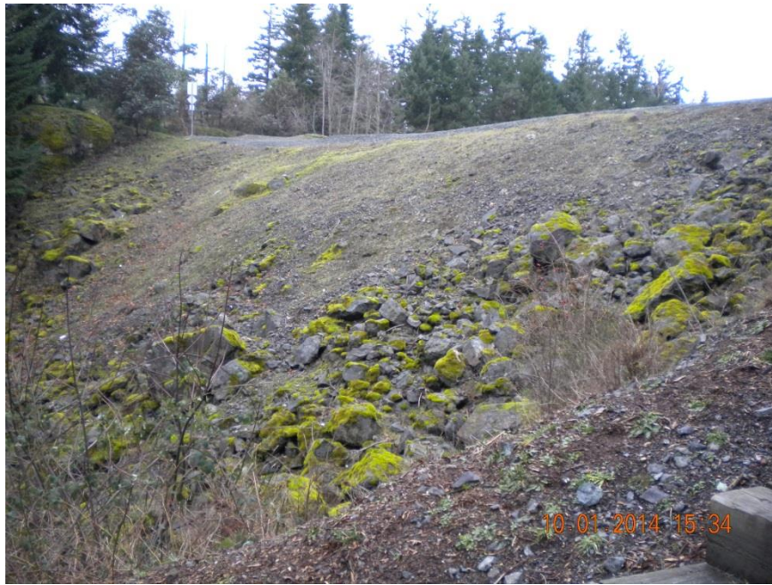
Photograph 3 – Upper portion of downstream slope of dam
