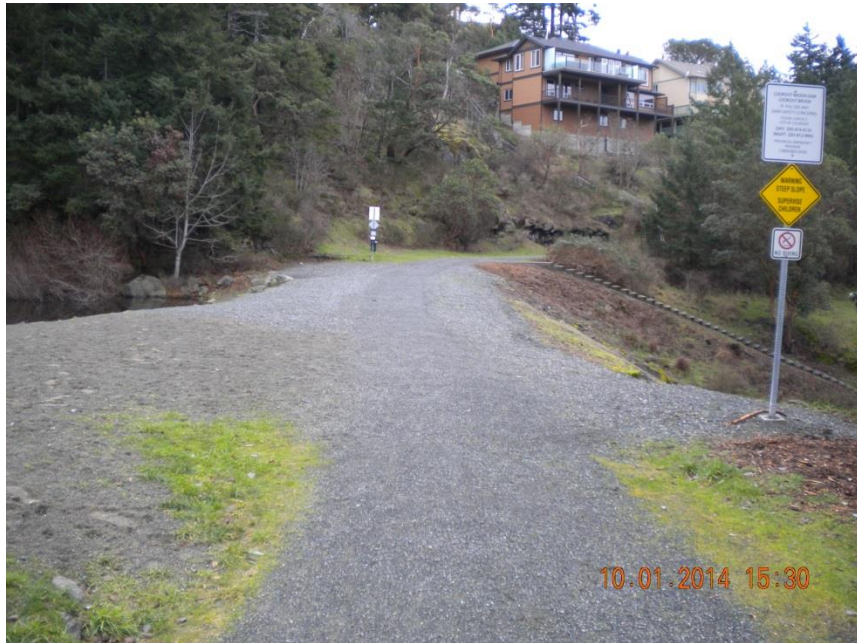
Photograph 1 – Crest of dam
