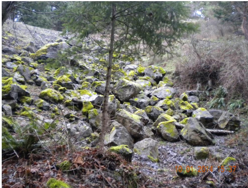
Photograph 4 – Lower portion of downstream slope of dam
