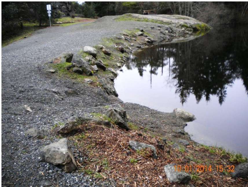
Photograph 2 – Upstream slope of dam
